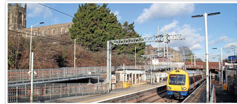
London Overground 172004 arrives at Upper Holloway with the late-running 1218 Barking-Gospel Oak on January 19. The route has been electrified ahead of the introduction of Class 710s from the spring. However, the wiring project has been delivered late. ANTONY GUPPY.
